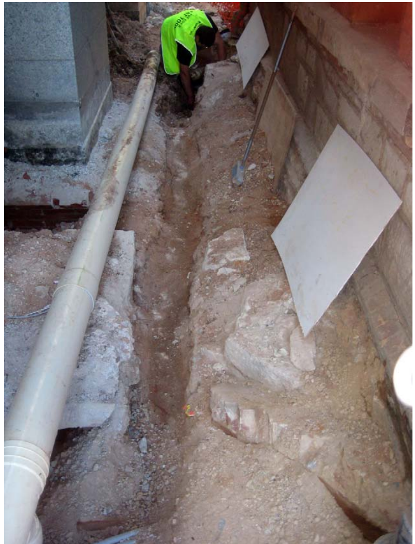
Fig.4 – Service excavations revealed the footings of the former east bay window which required diversion of the services (Swanbury Penglase 2012)
