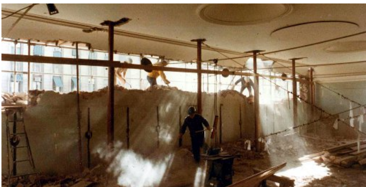
Fig.3 – Demolition in progress on the upper west wall of the former Legislative Council Chamber c1978, showing the extent of intervention carried out at the time ( History SA )
